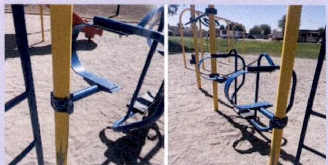
Playground was repaired.
