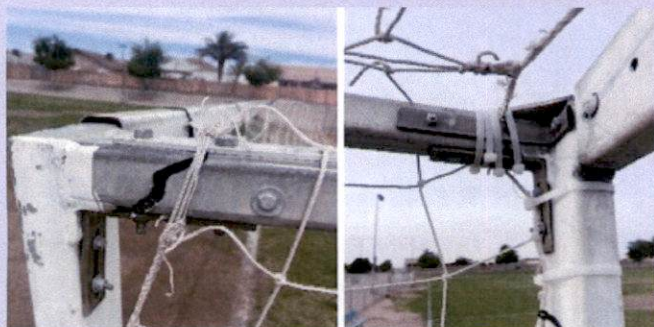
Soccer goals were repaired.
